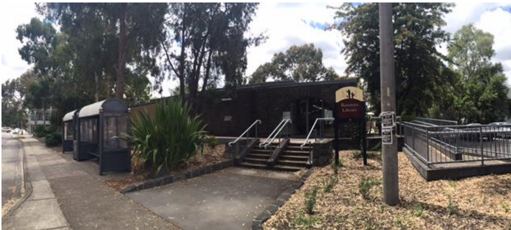
PICTURE 3 –STONE LIBRARY BUILDING AT THE SUBJECT SITE AND BUS STOPS ON TURNHAM AVENUE
