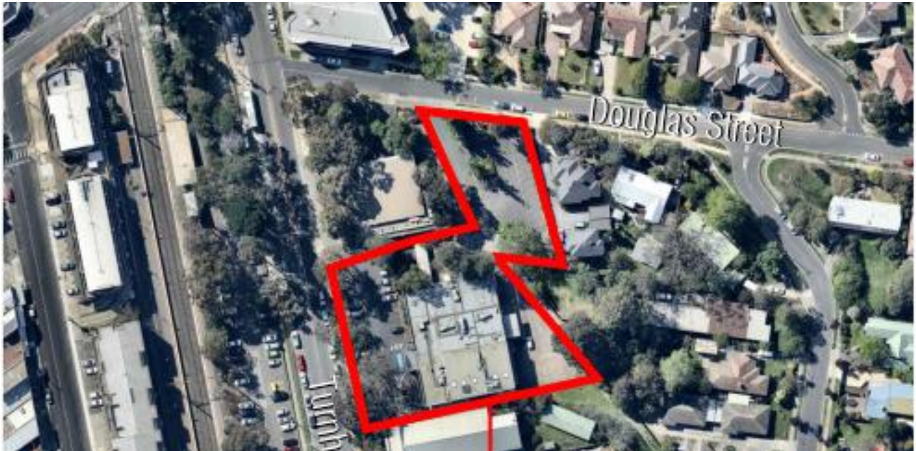
Fig 1. – Site aerial photograph
