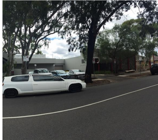
PICTURE 9 – INTERFACE TO THEATRE TO THE SOUTH OF THE SITE (RIGHT OF IMAGE)
