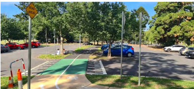
Figure 84 | New shared path and tree planting at Heidelberg Park
