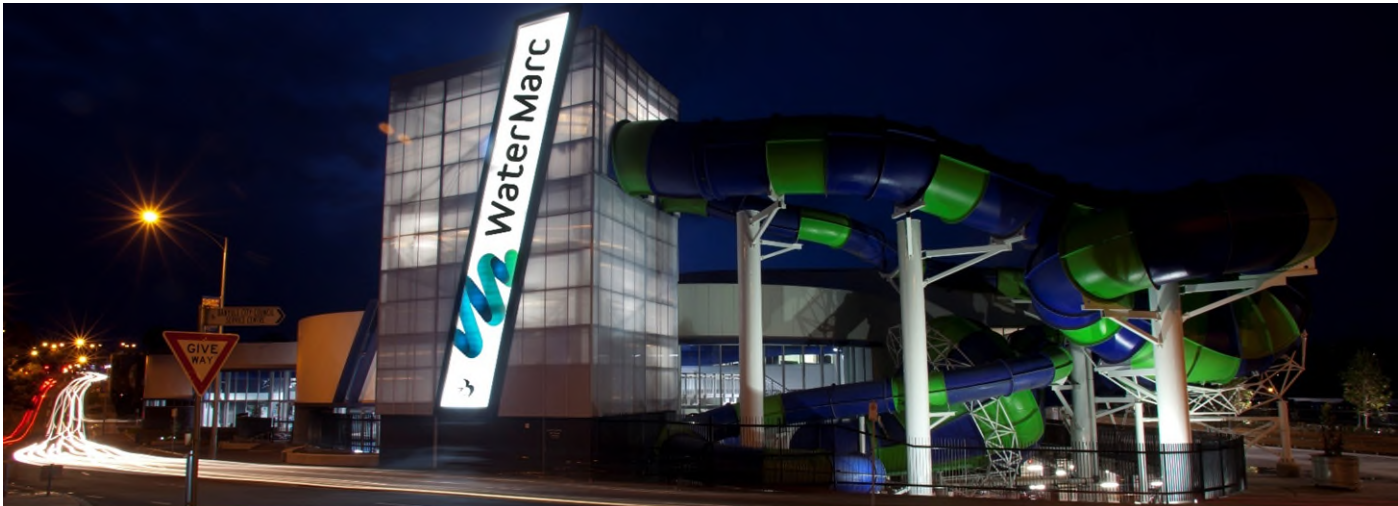
Figure 38 | Banyule Council’s main office alongside WaterMarc, right in the heart of Greensborough
