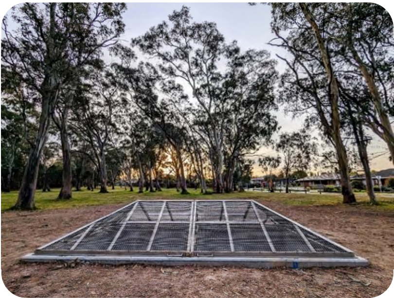
Figure 64 | Water sensitive urban design: stormwater litter trap, also known as gross pollutant trap, Greenwood Reserve, Bundoora
