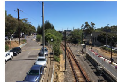
Figure 08 – View of railway tracks from pedestrian overpass looking north
