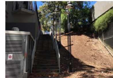
Figure 10 – View of staircases looking south towards 7 Flintoff Street carpark
