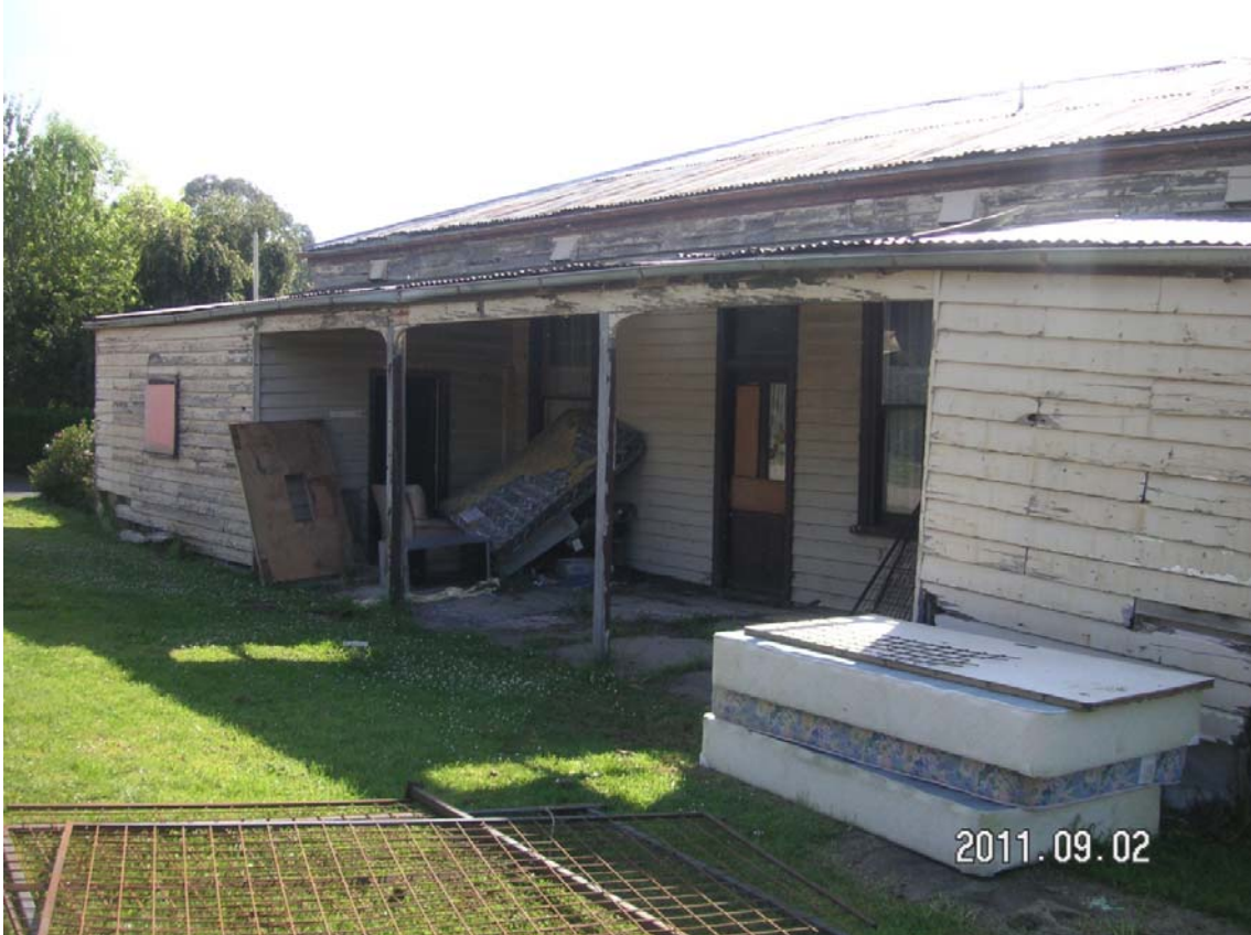
Figure 2: Rear of property showing recessed verandah
