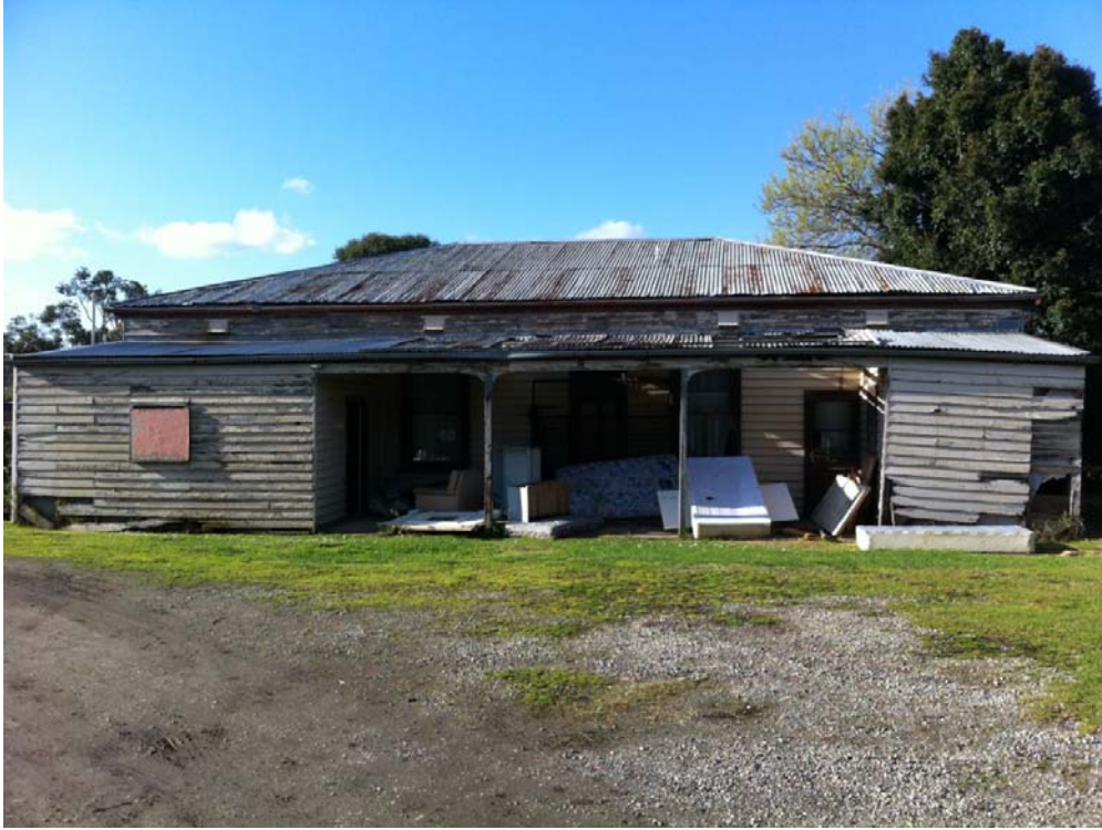
Rear Elevation – Saxam Homestead - July 2011
