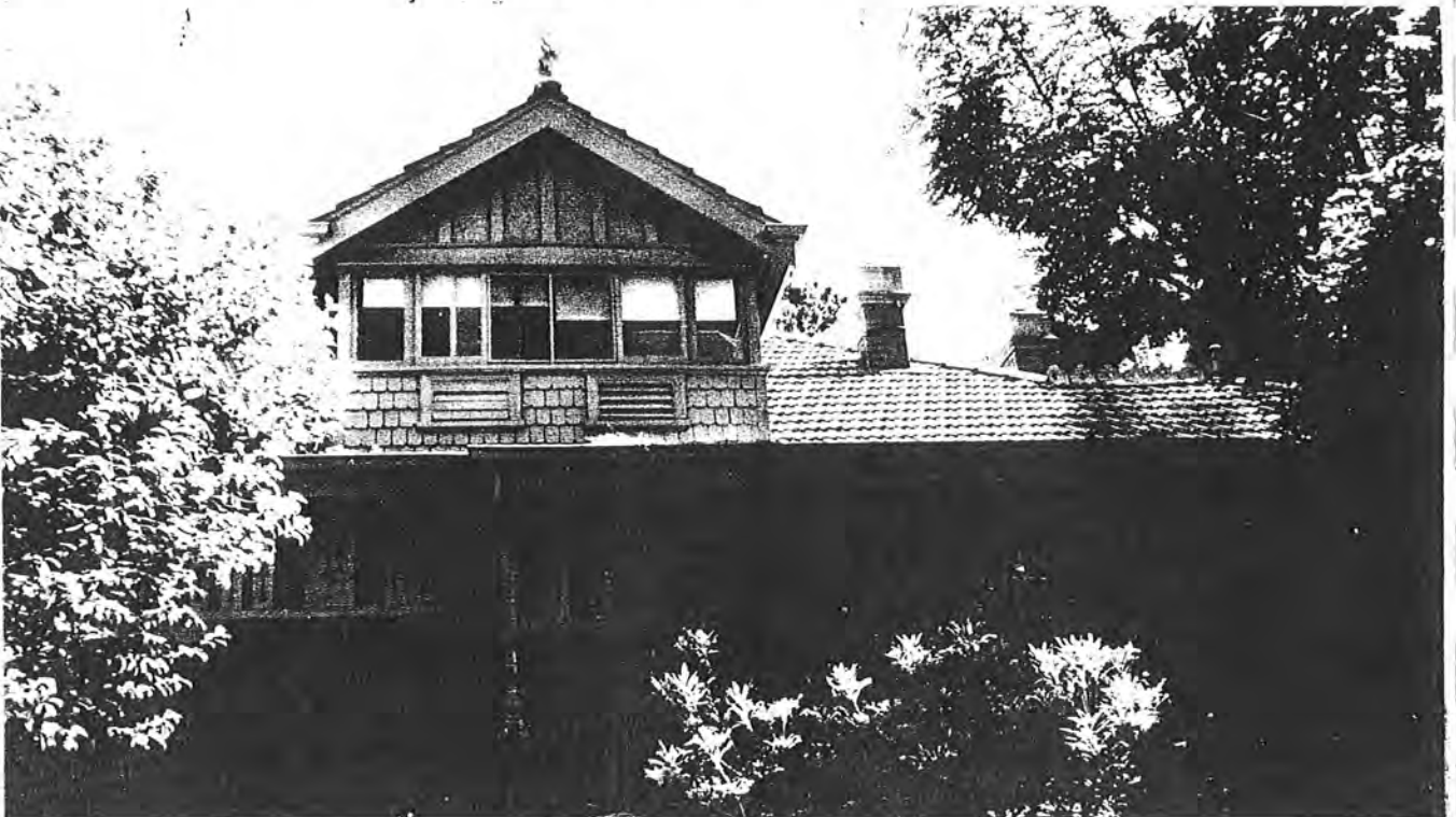
The Bent Tree, 47 Studley Road
