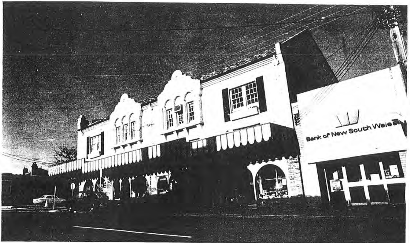
Shops and Dwellings, 218-224 Upper Heidelberg Road
