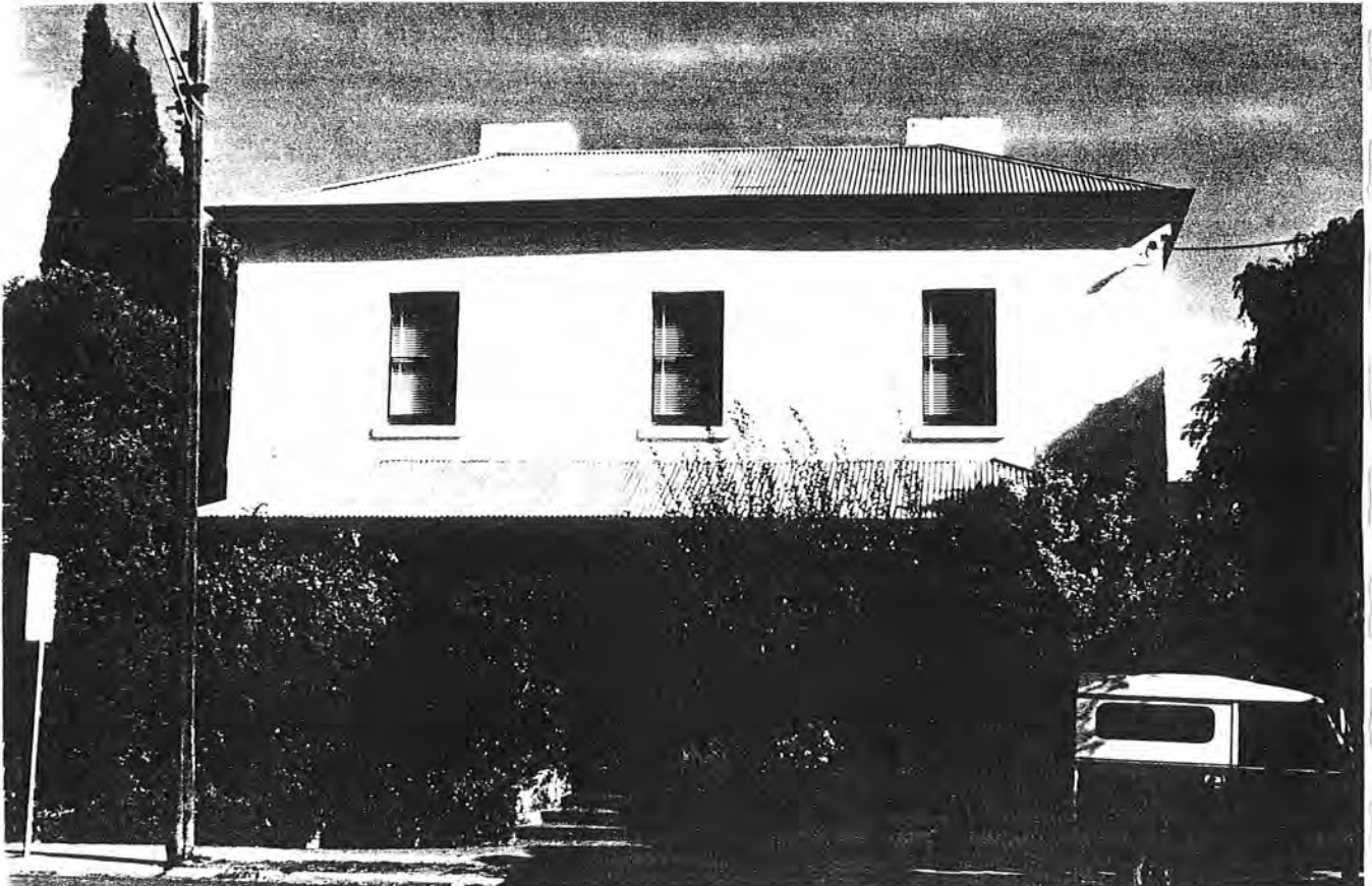
Former Darebin Bridge Hotel, 899 Heidelberg Road
