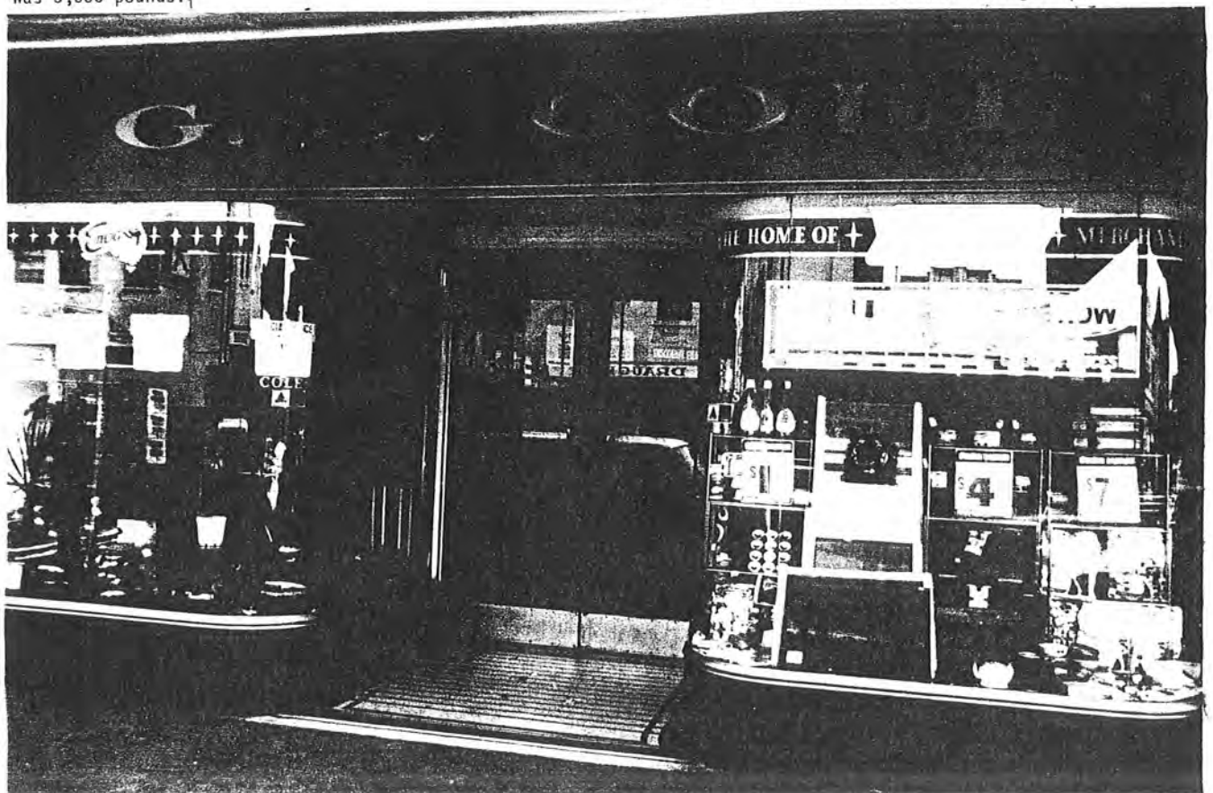
Coles Store, 115-117 Upper Heidelberg Road
