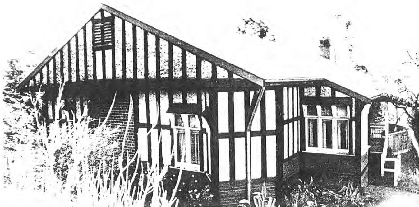
East View, 14 Martin Street
