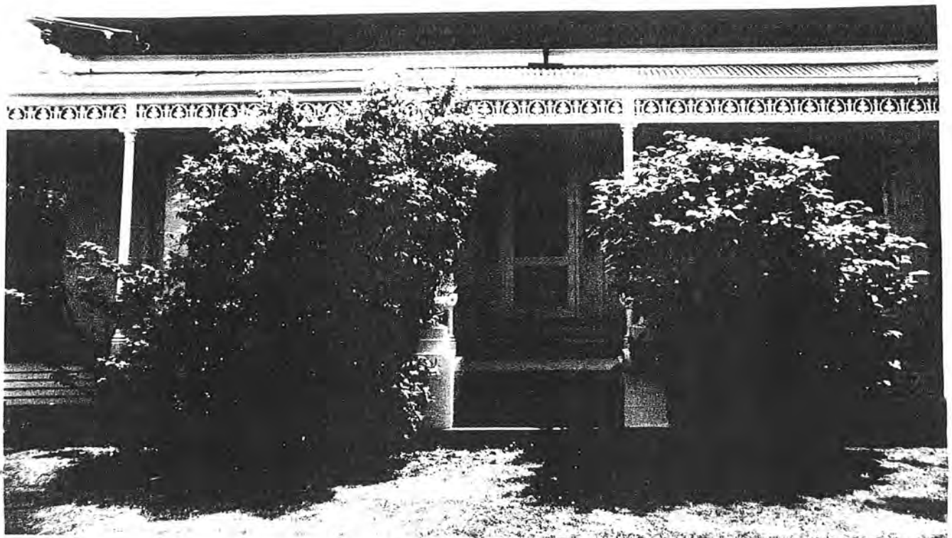
A view of Cintra's eastern facade
