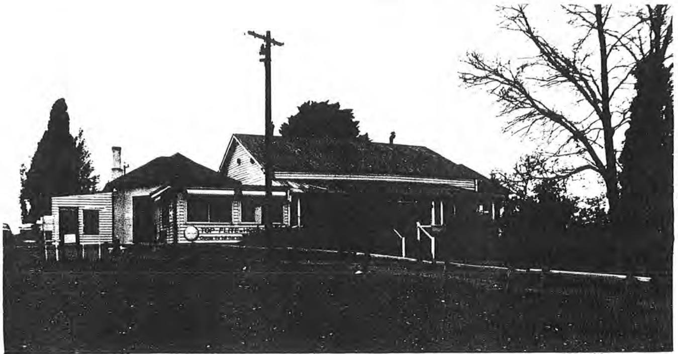
Original masonry bays flank an altered or replaced timber centre and are themselves flanked by sundry and damaging additions
