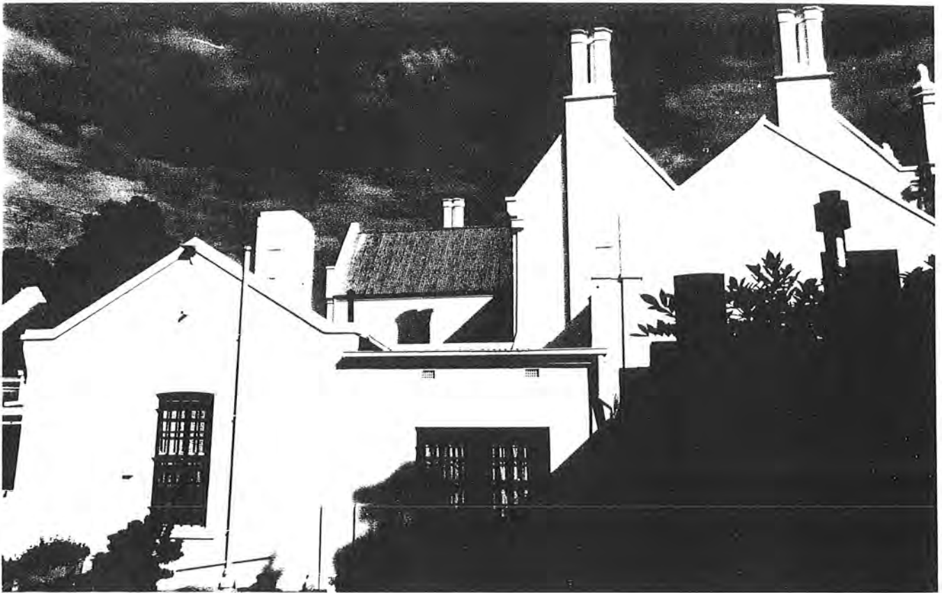
A view of the northern elevation which was possibly the earliest part of the Banyule complex c1843
