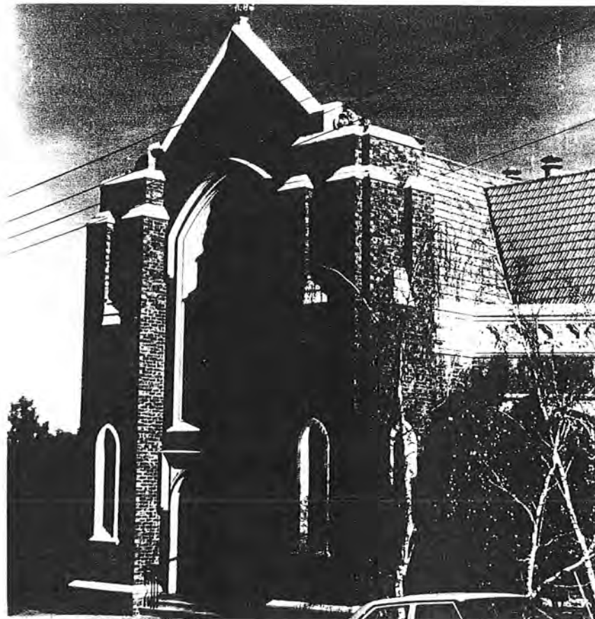
Former Knox Presbyterian Church, Noel Street
