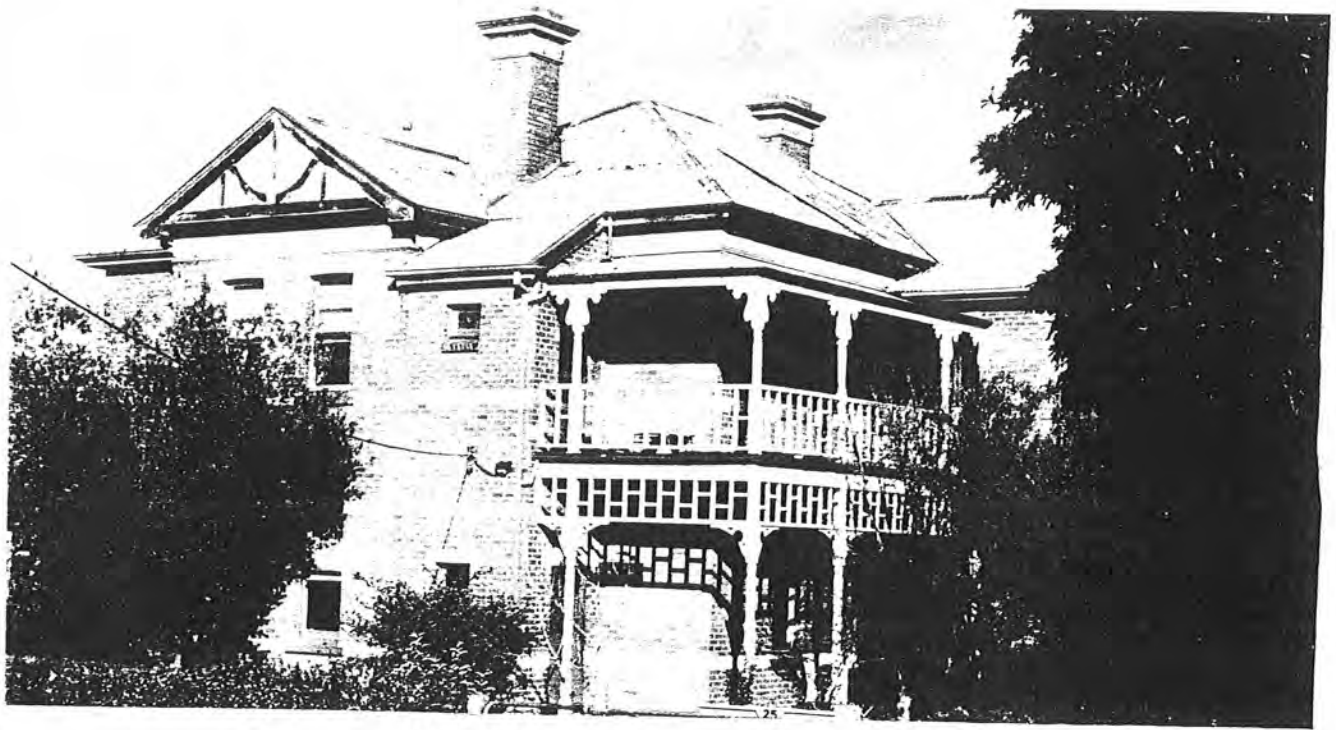
Kennington Flats, 25 Rose Street
