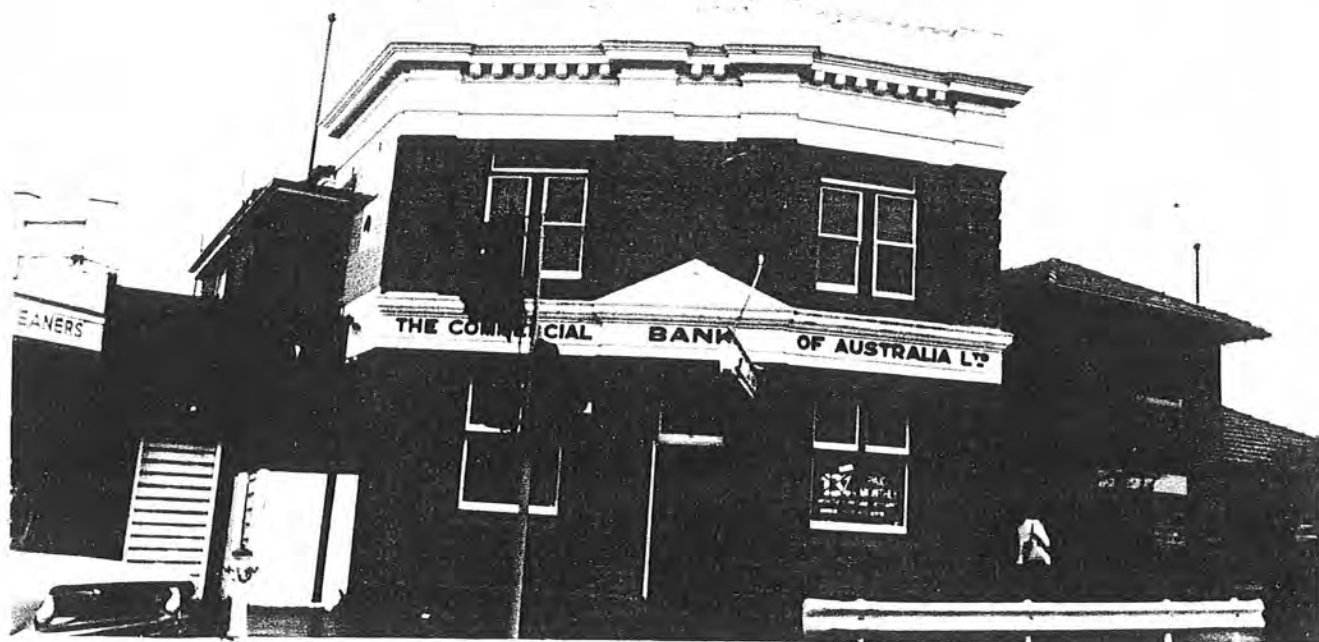
Commercial Bank of Australia, 147 Upper Heidelberg Road
