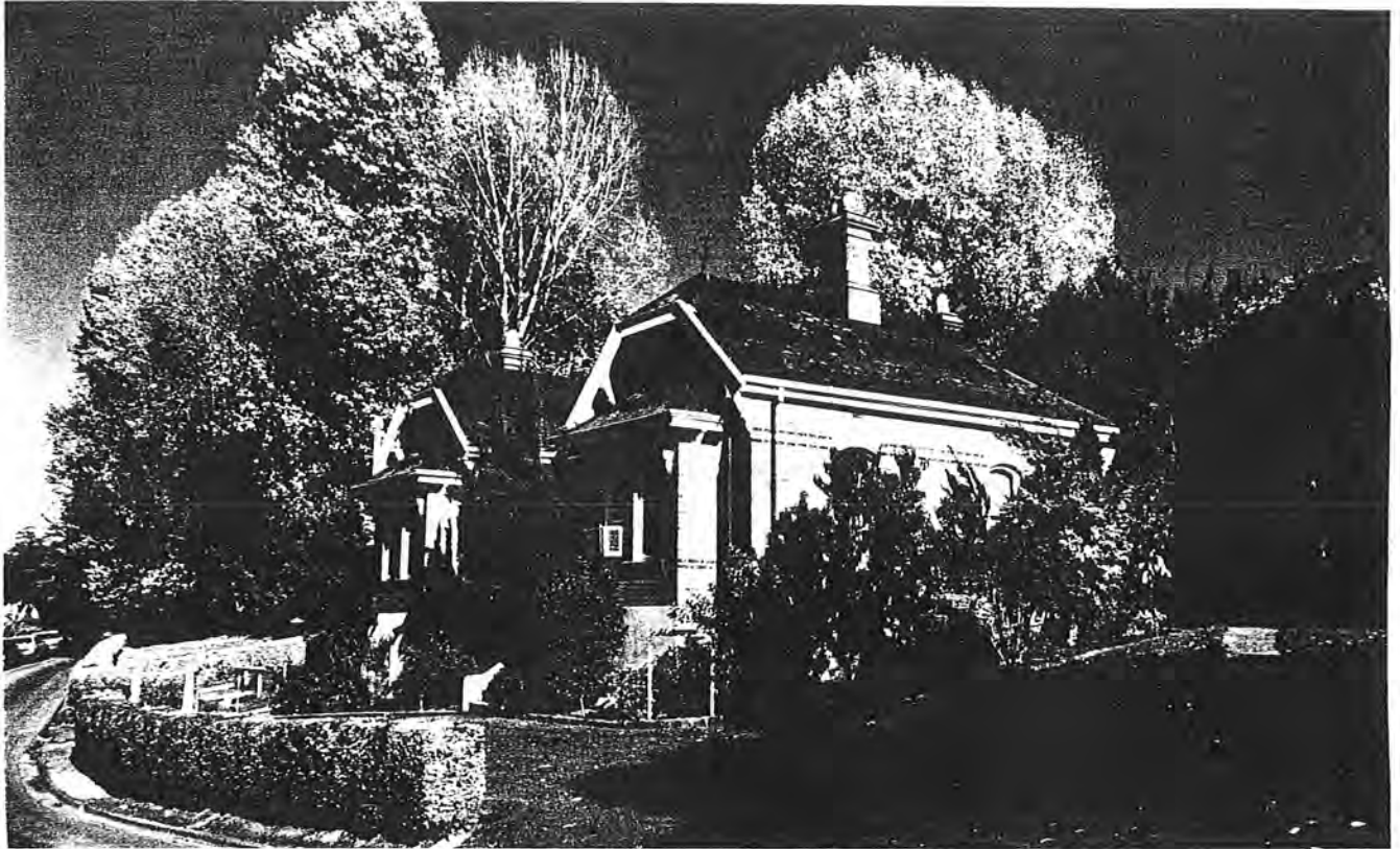
The former Lodge, Austin Hospital
