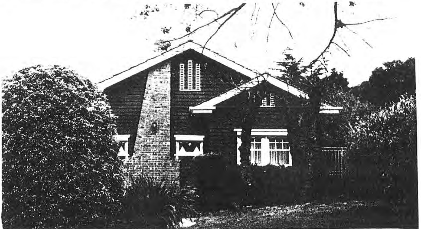
House, 6 Glenard Drive
